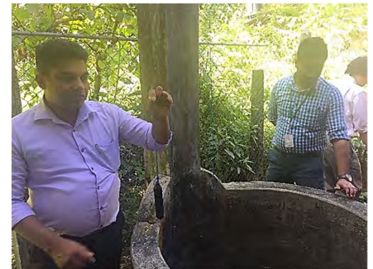
Installation of data logger 5
