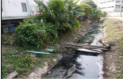
Small pipes discharging gray water from households, hotels and restaurants along the right bank in the upper half of this stretch
