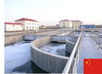
Urumqi (10 thousands m 3 /day: Oxidation Ditch)
