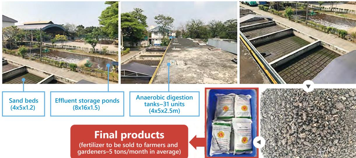
Figure 7. Nonthaburi city faecal sludge treatment plan and fertilizer produced as final product
