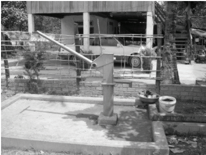
Ground Water from a Hand Pump
