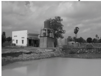
Water Treatment System
