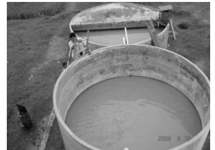
C.F.S. Tank and Slow Sand Filter
