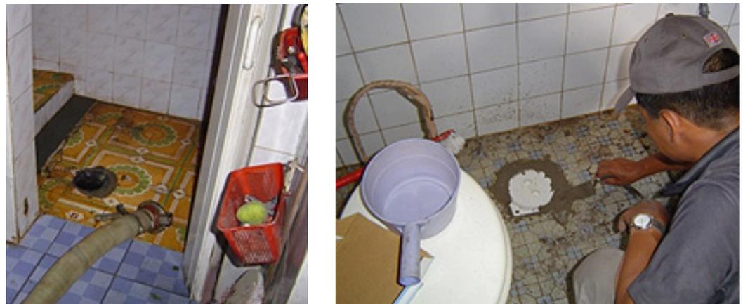
Worker installing plastic cover to the access hole after emptying septage in Hai Phong city
