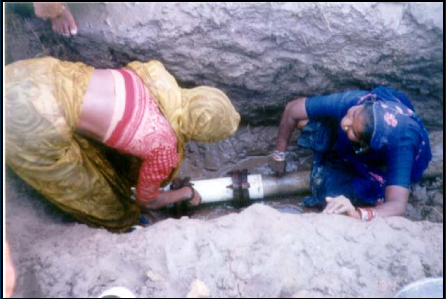
SEWA 2003 – pipeline maintenance by women
