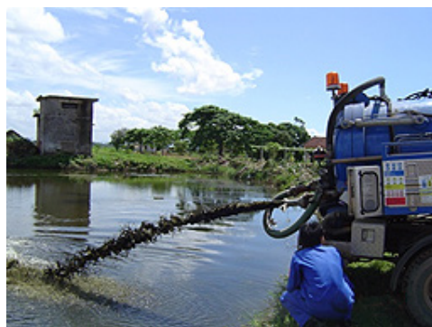
Direct discharge of septage into fish pond in the peri-urban area Source: Author
