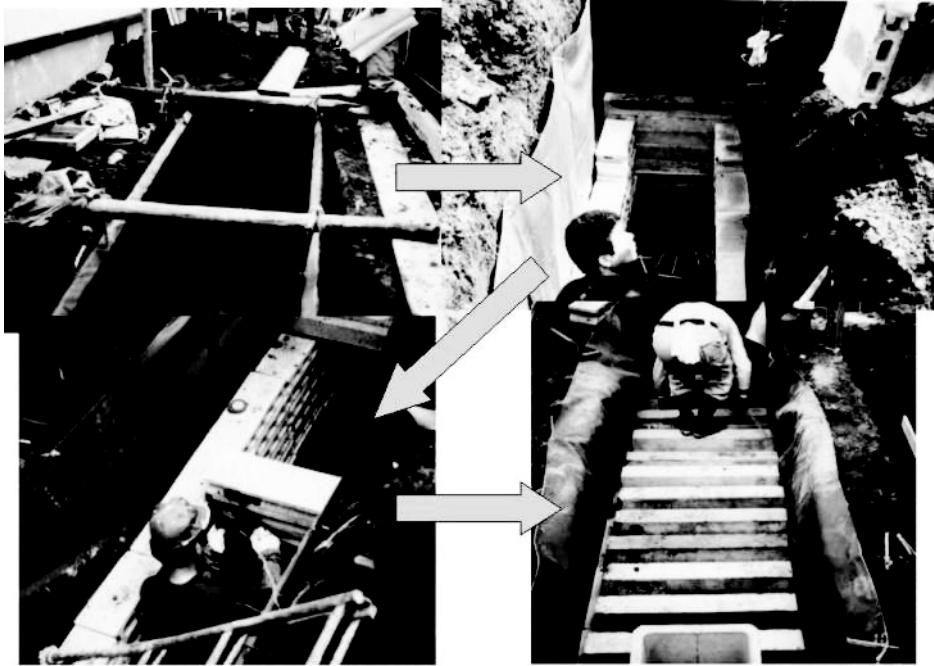
Figure 2. The construction status of the low cost facility.
