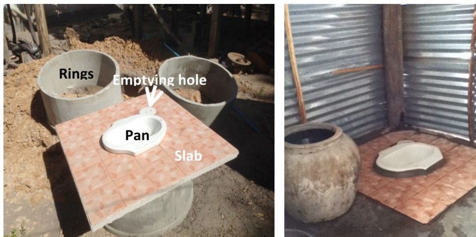
Figure 1-5.1 Pour-flush Toilet [Water and Sanitation Program, 2016]
