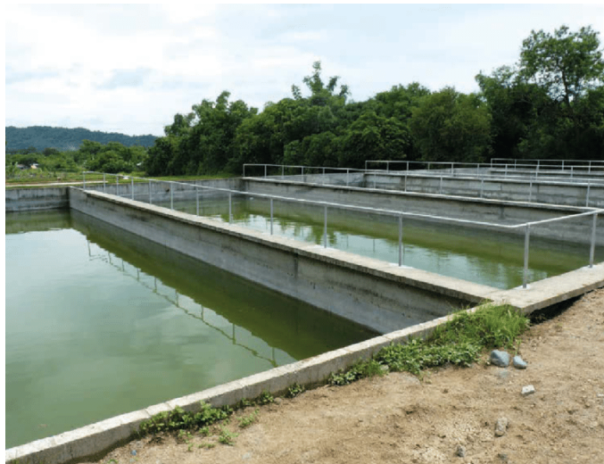
Figure 3.4-8. Faecal Sludge Lagoon System, San Fernando City, Philippines (Strande, Ronteltap, & Brdjanovic, 2014)
